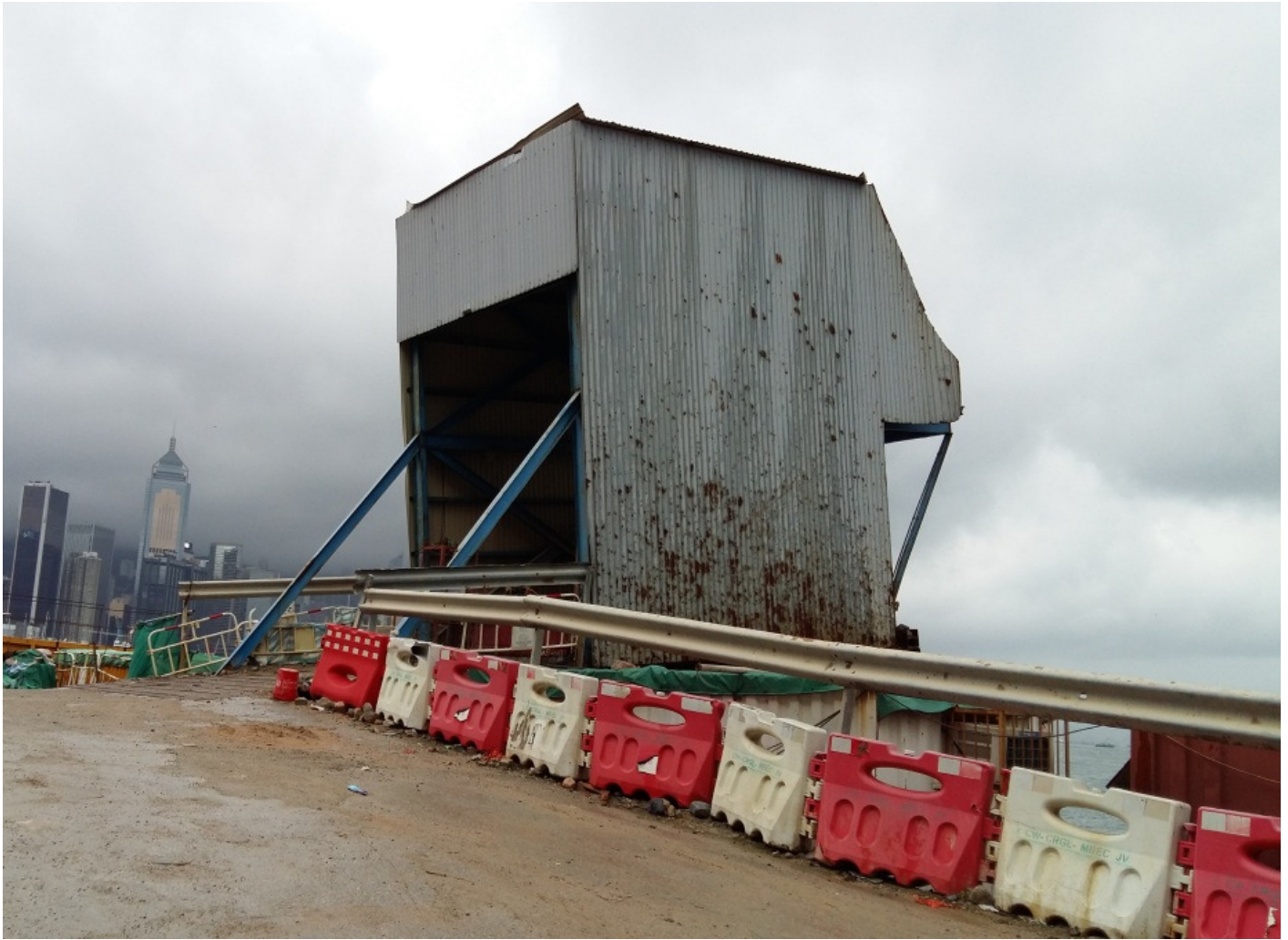
Photo No. 1 – General Views of Temporary Jetty
